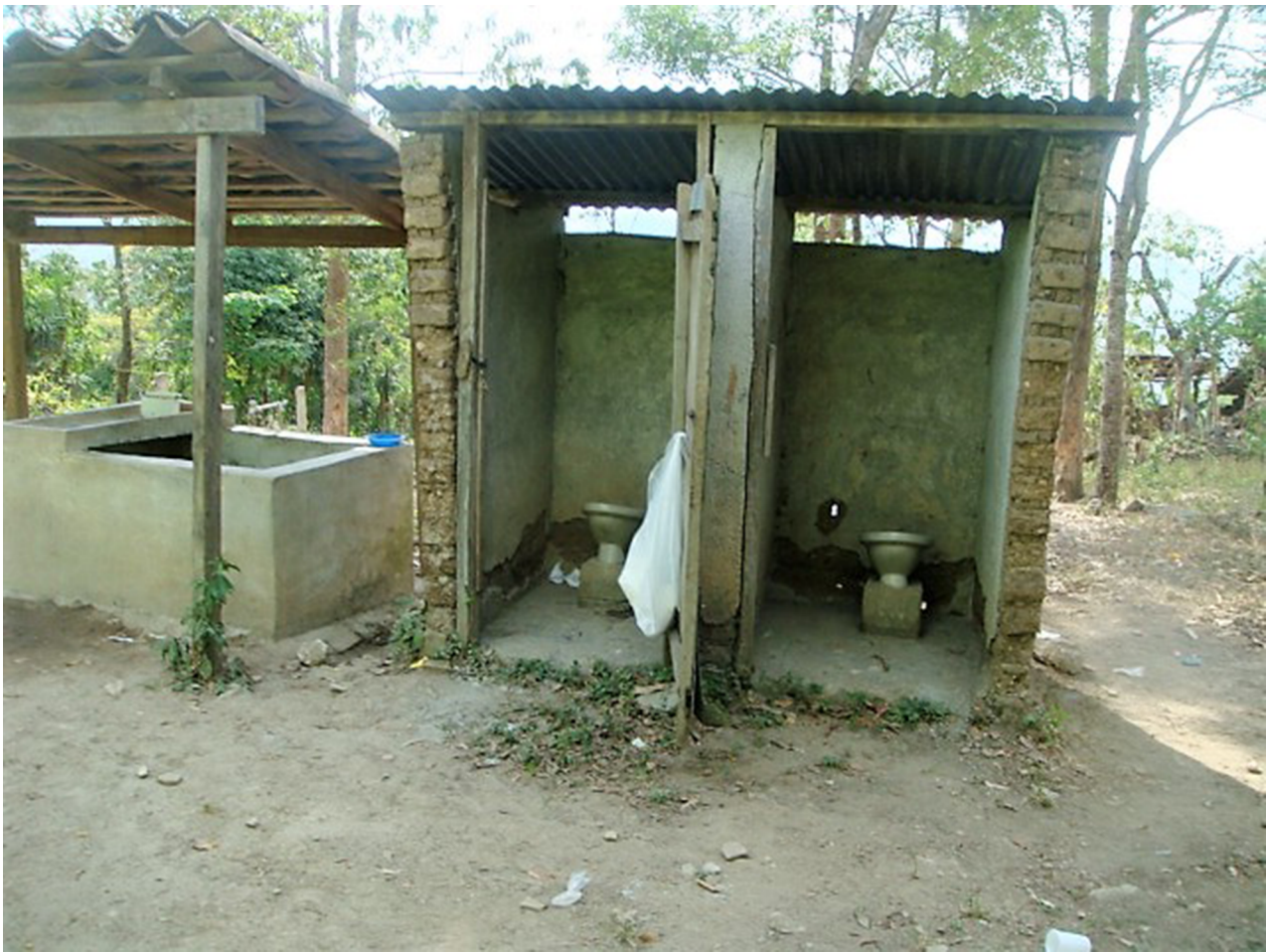
Figure 2 An open and uncovered water source within meters of the village latrine or outhouse facility.
